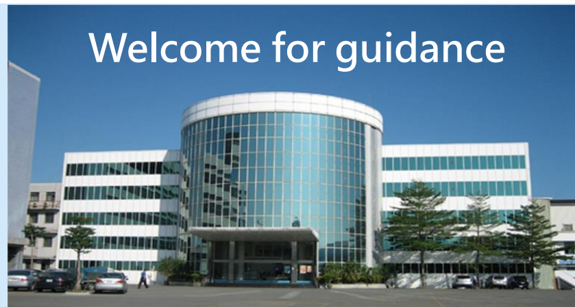
▲ Taiwan Exhibition Center in HCG 3rd Factory
